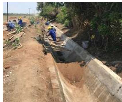
Rehabilitation of the irrigation system
