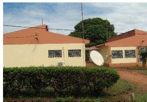
Rehabilitated Administration block at Sussundenga
