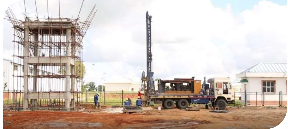
Construction of water tank and water hole
