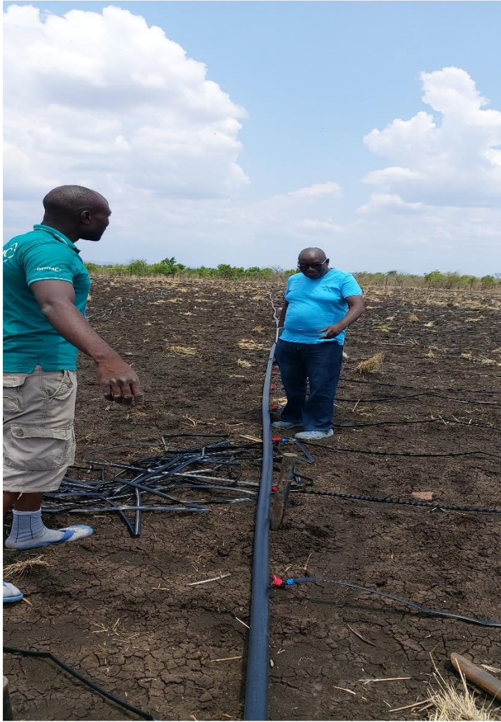
Figure 3: Infrastructure completed in Zambia
