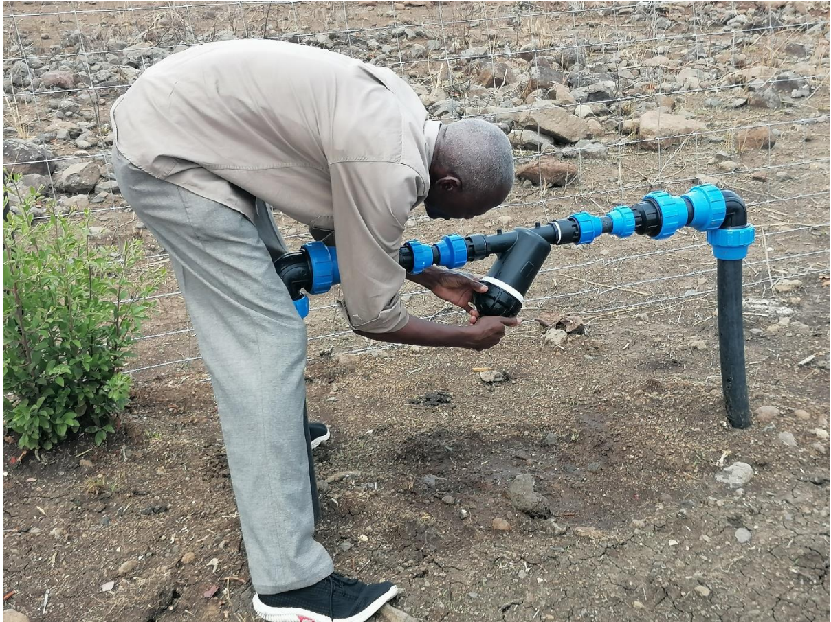
Figure 5: Irrigation Engineer inspect the water filter at Katapazi Irrigation Scheme
