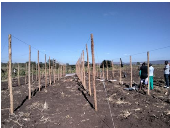
Figure 3: Construction of a greenhouse at the project site in Mozambique.
