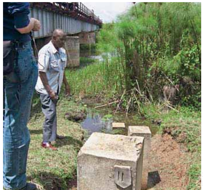
Water level indicator for flood monitoring
