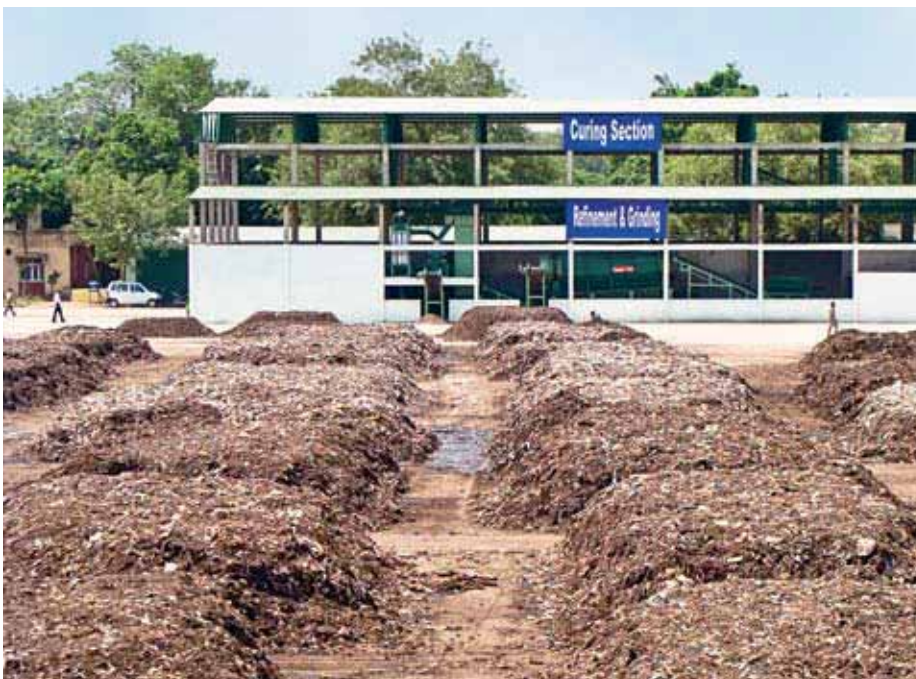
Municipal solid waste composting in the industrial area of New Delhi
